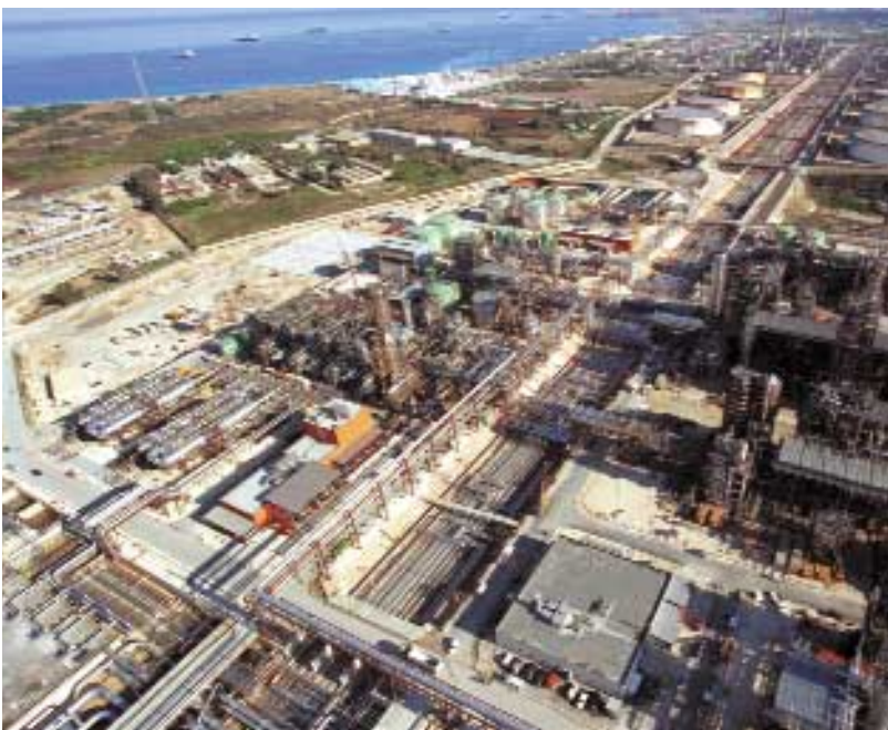
General overview of the complex taken from the top of the 130m tall stack.
