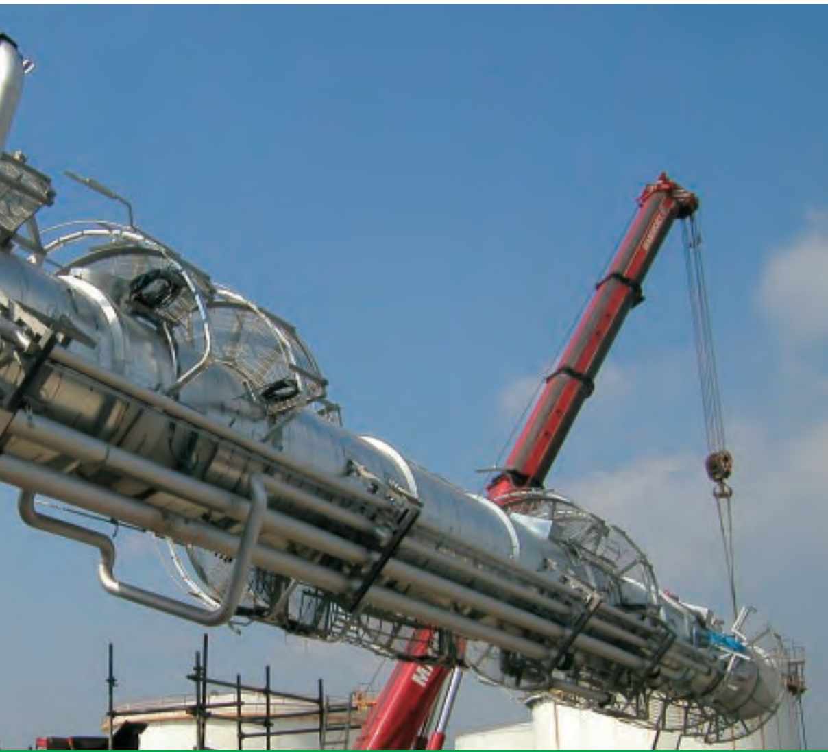
Unit 36 fractionator heavy lift almost complete.
