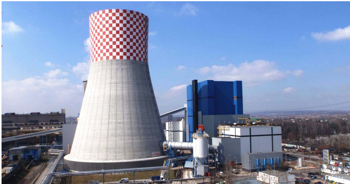
Figure 1 New 460 MW e Łagisza CFB OTU Unit
