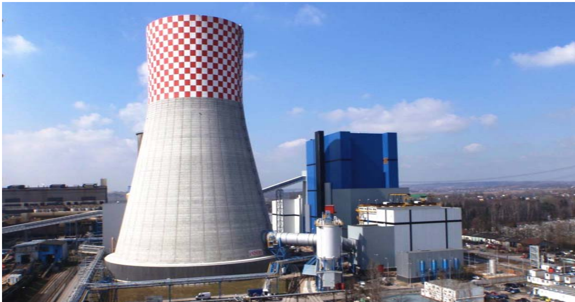
Figure 1 New 460 MW e Łagisza CFB OTU Unit
