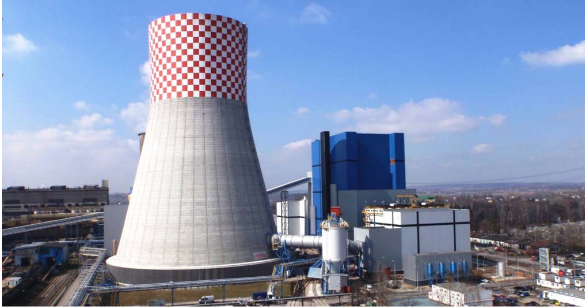
Figure 1 New 460 MW e Lagisza CFB OTU Unit
