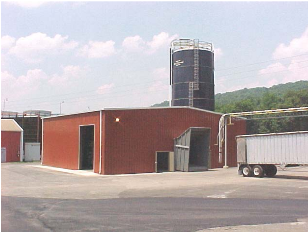
Figure 1. Cofiring Installation at Albright Generating Station. Housed in the Structure are the Fuel Receiving, Screening, Metering, and Pneumatic Transport Systems.
