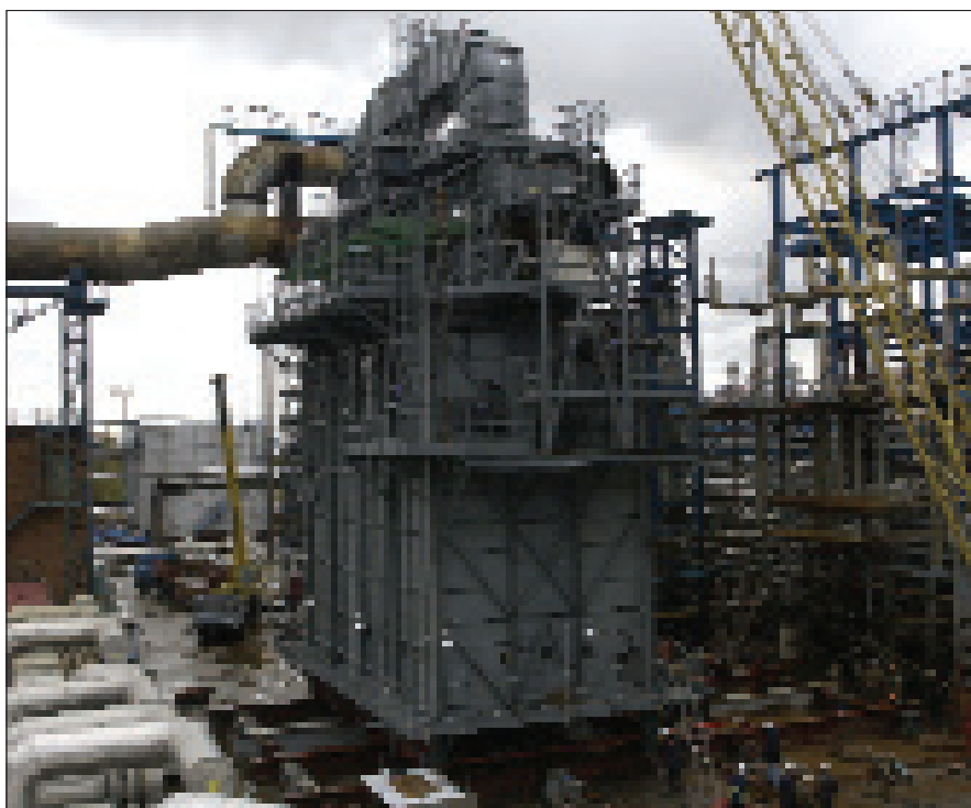
Figure 7 Furnace installation prior to startup
