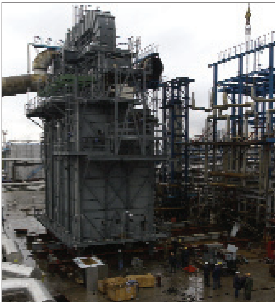
Figure 6 Final preparations to new furnace
