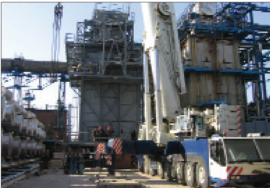
Figures 1 to 3 On-site heater assembly
